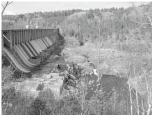
Figure 51. McConnell Lake Dam (2000).
