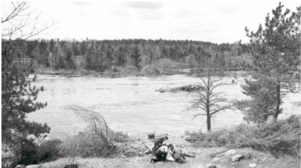
Figure 35. Historical view of the rapids where Chenaux Generating Station was constructed. View is from the east on Limerick Island (OHSC Archive Neg. No. 1947).
