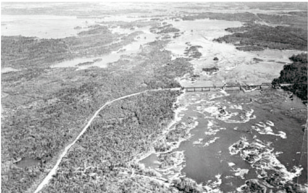
Figure 23. Aerial view of Chats Rapids and Chats Falls from upstream, 1920 (National Archives of Canada C22209).
