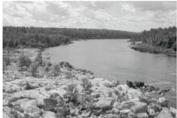
Figure 36. The overflow channel constructed through Limerick Island (2000).
