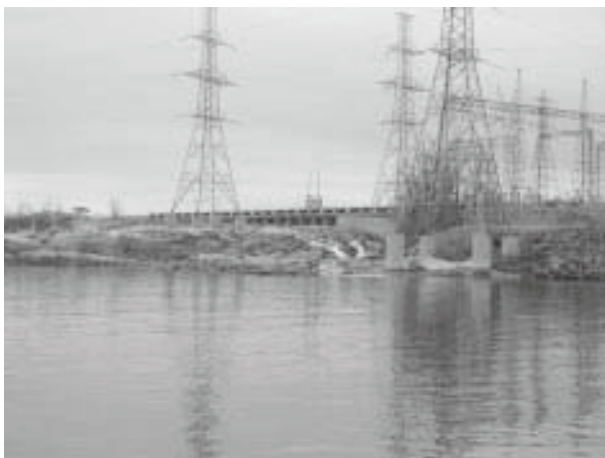
Figure 27. Sluice gates and structures at Horseshoe Chute, 2000.
