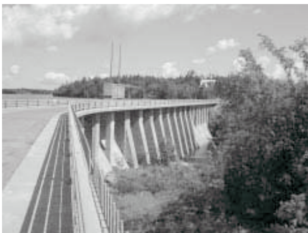
Figure 39. The dam constructed at Portage du Fort (2000).
