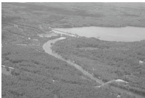
Figure 52. Des Joachims Dam and tailrace channel (1997).
