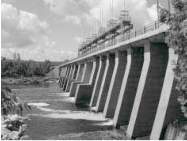
Figure 37. Limerick Island control structure (2000).
