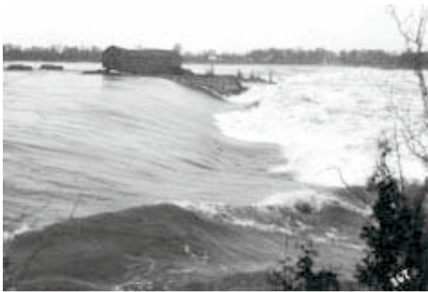
Figure 6. Carillon Dam during the spring flood of 1908 (National Archives of Canada PA 85631).
