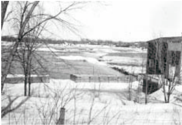
Figure 5. Old crib dam at the Carillon site (Quebec Hydro Archives).
