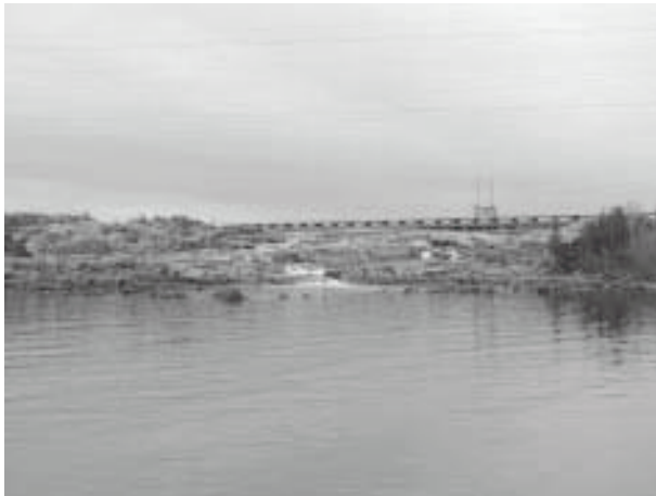
Figure 26. Sluice gates and ancient waterway at Ragged Chute, 2000.
