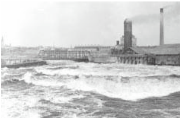
Figure 14. Chaudière Falls during high water in 1909 (National Archives of Canada PA 9415).
