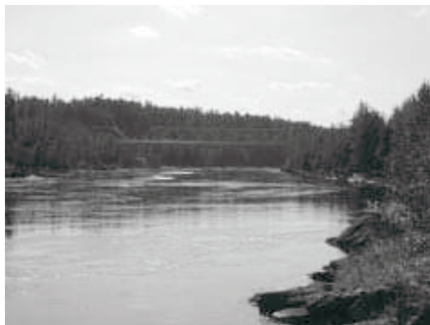
Figure 53. Swift current in the tailrace of Des Joachims Dam (2000).
