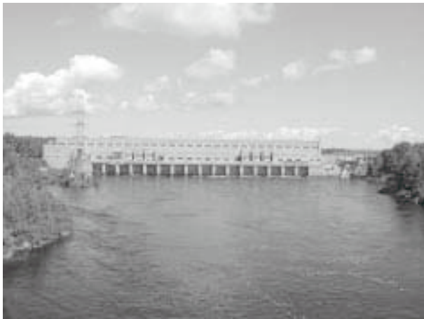
Figure 38. Cheneaux Generating Station (2000).
